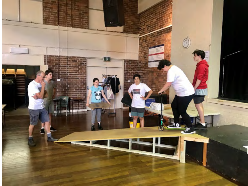
Bob Herman asking students to test the ramps during construction.
